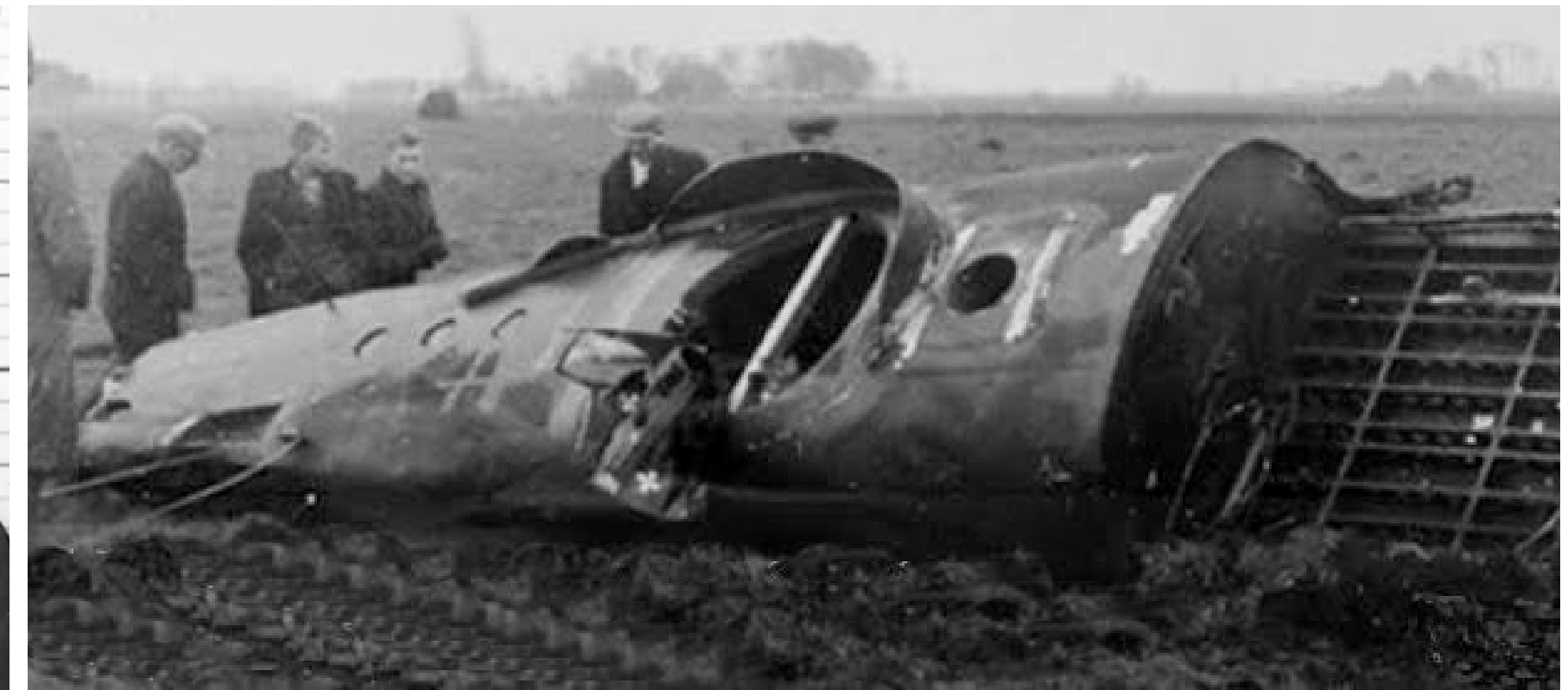
Dutch citizens come to look at the wrecked fuselage of Lancaster JB280 lying in a farm field near the town of Nieuw-Schoonebeek, Drenthe, Netherlands. The framework on the right of the fuselage is the floor above the bomb bay with doors gone. The faring around the hole in the centre of the fuselage section is for the H2S Radar, the antenna housing having been destroyed. These wrecks would soon be loaded onto trucks and driven away to be melted down for German production. Photo via drentheindeoorlog.nl
